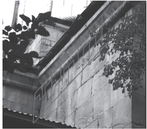
Fig. 1, 1-3. Lower wall of the southern arm of the main temple of the Georgian monastery Khakhuli, located in Turkey's north-east in the village Bagbash in Erzurum Province, has an anti-seismic effect belt. Stones are cut in such way that they do not slip. Due to the use of such method the church is preserved in its original form. (photo G. Bagrationi)
