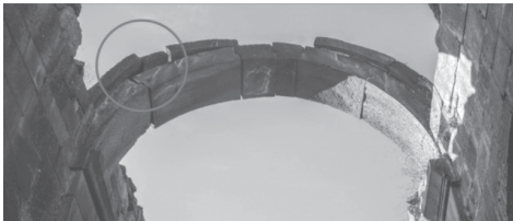
Fig. 2, 1-2. Builder of the Georgian Church Akori in Lore district (Armenia) faced the same problem. He used the same anti-seismic method to preserve the building. The stones are mounted with rectangular strips of arched beams so that their separation is much more complicated than that of the usual arch. (photo G. Bagrationi)
