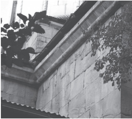
Fig. 1, 1-3. Lower wall of the southern arm of the main temple of the Georgian monastery Khakhuli, located in Turkey's north-east in the village Bagbash in Erzurum Province, has an anti-seismic effect belt. Stones are cut in such way that they do not slip. Due to the use of such method the church is preserved in its original form. (photo G. Bagrationi)
