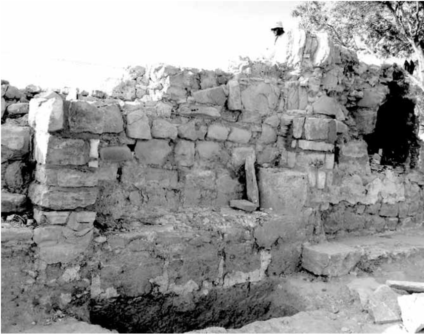
The partial restoration of the Northern wall and the pilasters of Alaminos church
